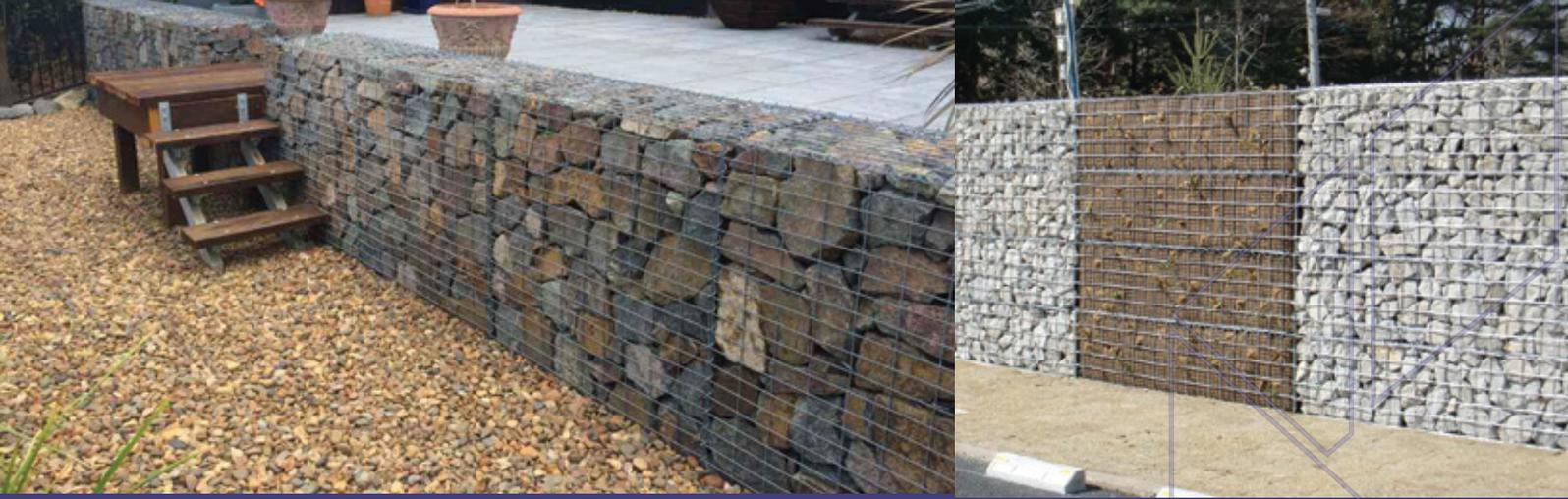
Welded mesh gabions are a valid and effective technical solution in the design, construction and maintenance of a variety of civil structures. They can provide an effective, economical and environmentally acceptable solution to a range of civil engineering problems. Welded mesh gabions are more aesthetically pleasing, quicker and cheaper to install than woven mesh gabions.
